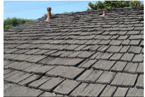
Front left view of the roof.
