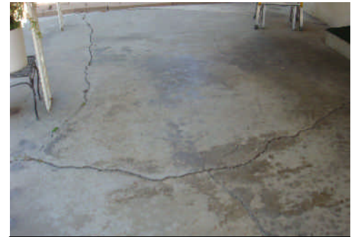
Expansion joints were not installed.
