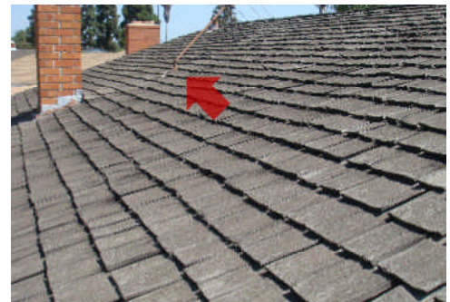
Rear view of the roof.
