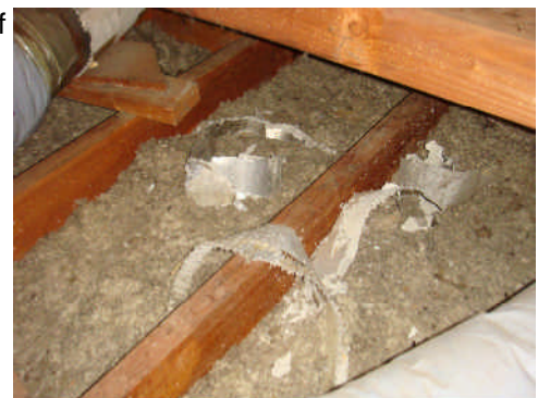
Return air duct chase not sealed/insulated
