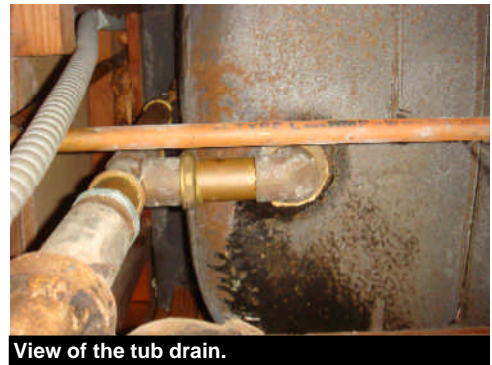
View of the tub drain.
