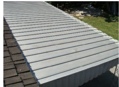
Expansion joints were not installed.
