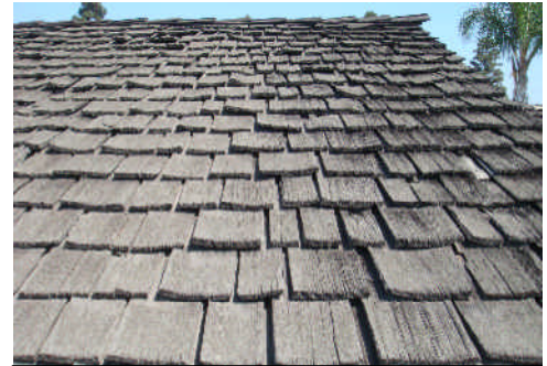
Front south facing side.
