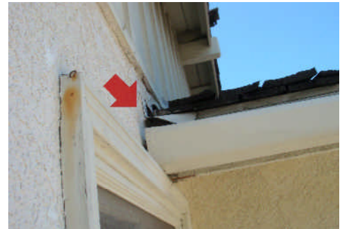
Install kick-out flashing.
