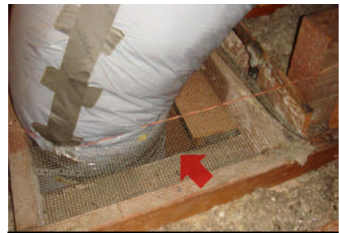
Return air duct chase not sealed/insulated
