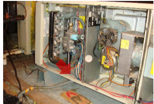
Gas flex connector in contact with housing
